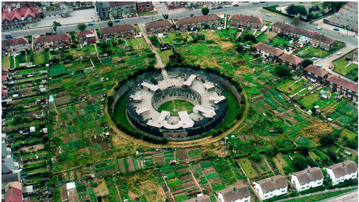
Fig. 37 Aerial view of the Harwich Redoubt
