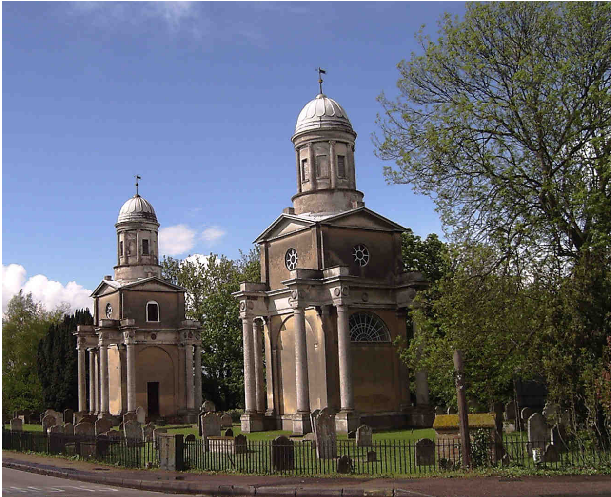
Fig. 64 The Mistley towers are all that remain of the church designed by the architect Robert Adam.
