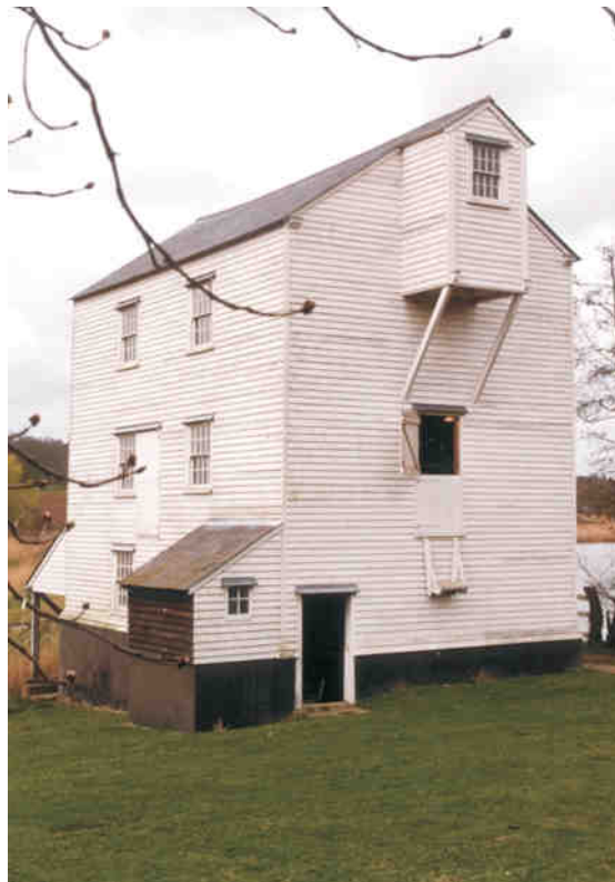
Fig. 69 The 19 th century timber-framed tide mill at Thorrington
