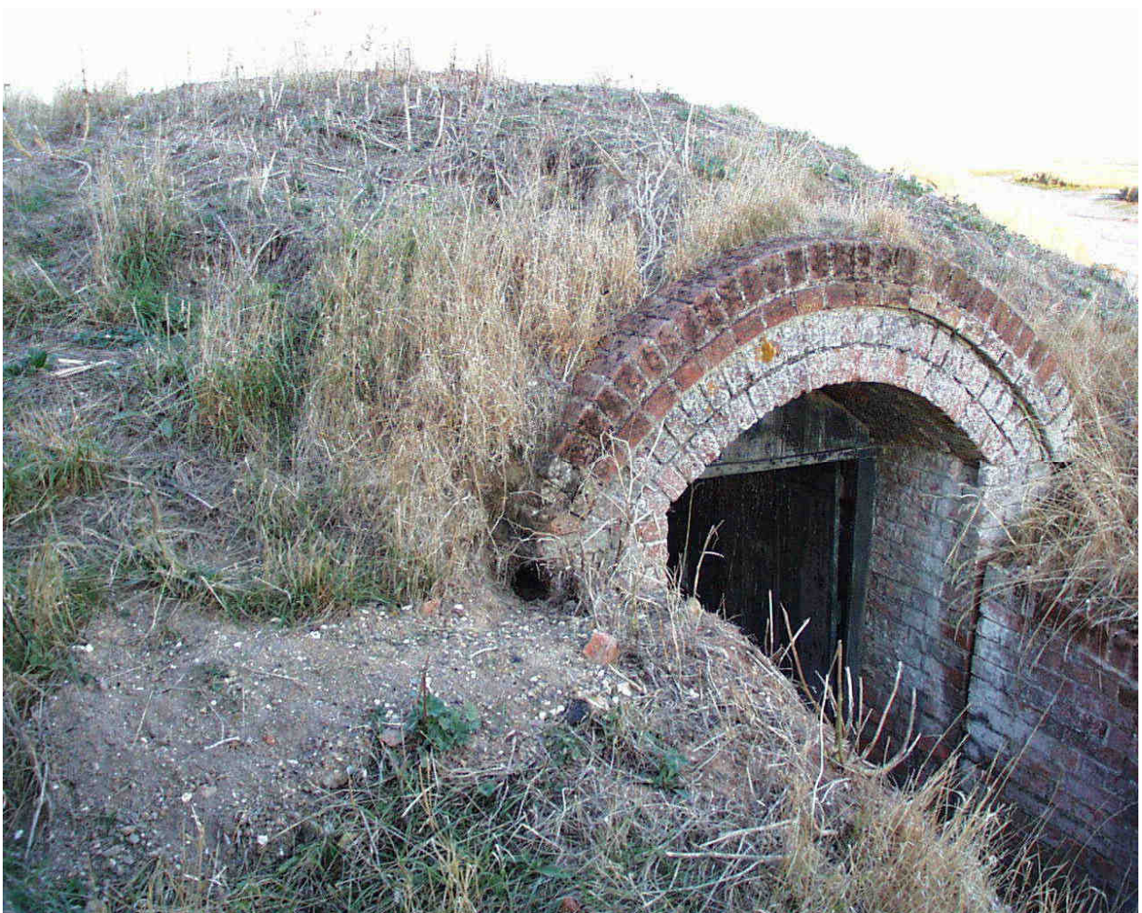
Fig. 16 The 19 th century Lime Kiln at Beaumont Quay
