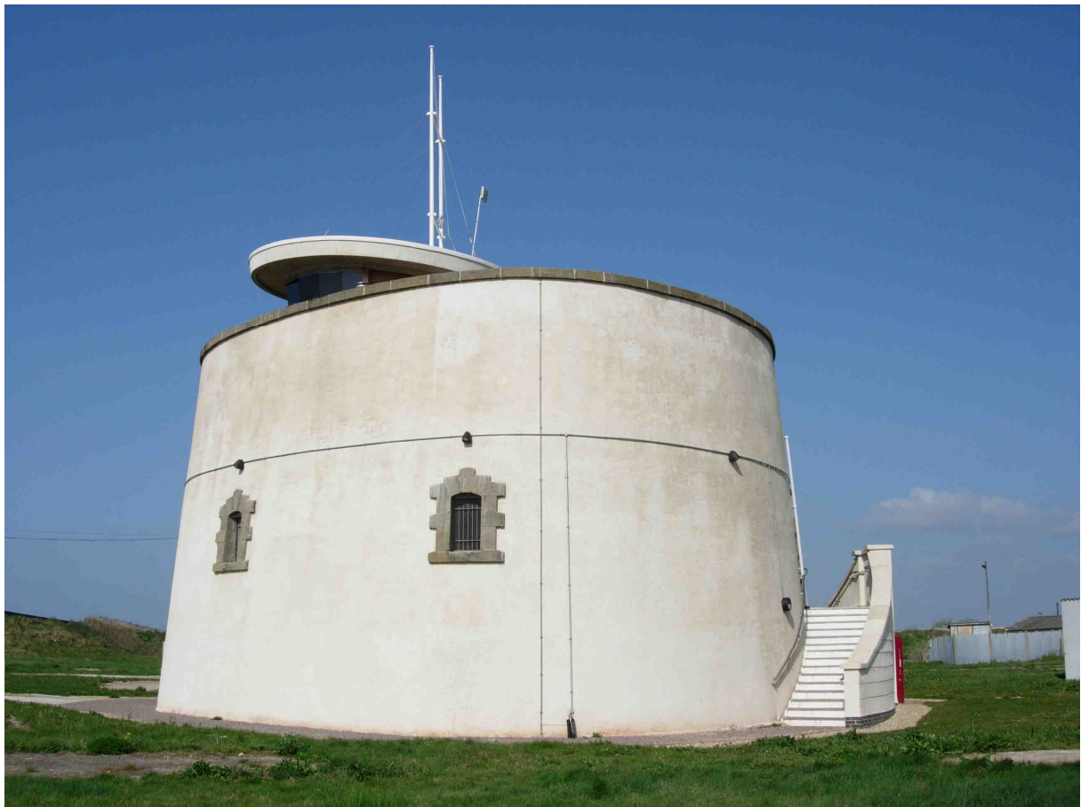
Fig. 21 Restored Martello Tower, Clacton
